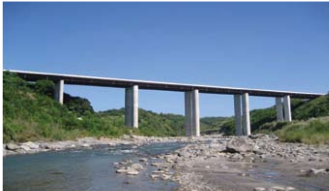
Sacobia-Bamban Main bridge, longest bridge at 1.16 km.
